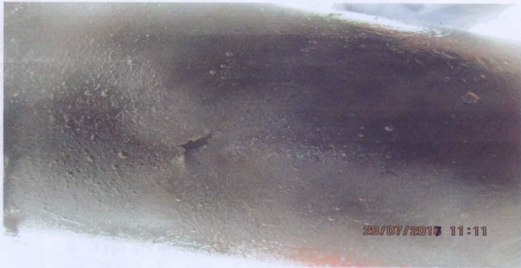
Spill point (a tear @ 6 o' clock position)
